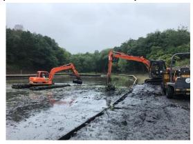
Once the barrier is in place the water from the moved silt will run back into the pond waters, the silt will eventually dry out and the bank will be planted with suitable vegetation.
